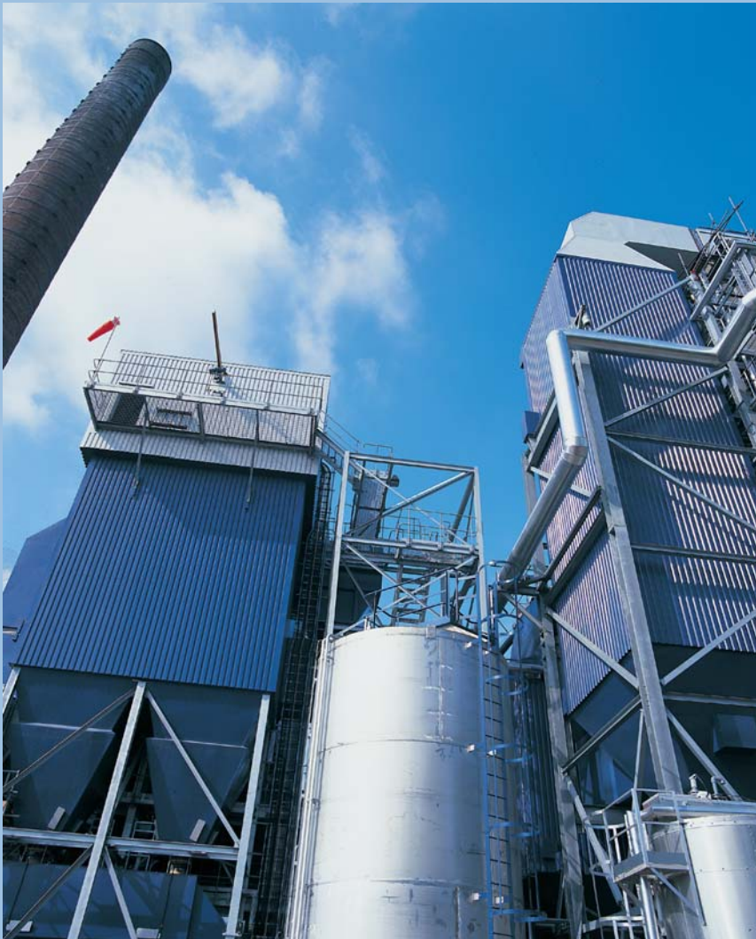
Bolton Thermal Recovery Facility
